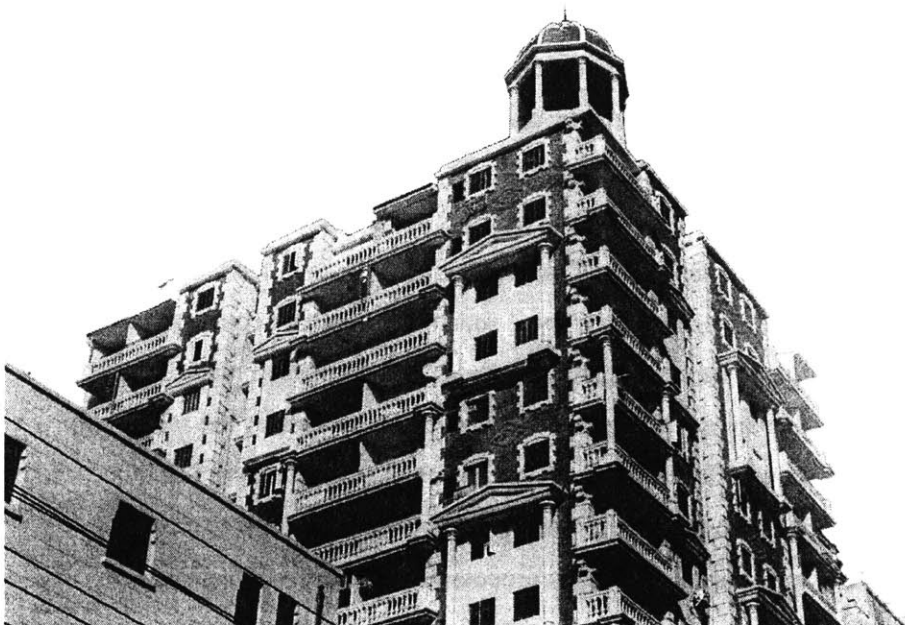
Figure 15. Historicism in a new apartment building
